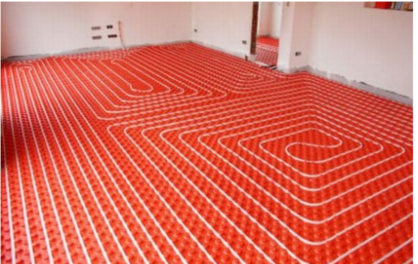
Pannelli radianti a pavimento Floor radiant panels
