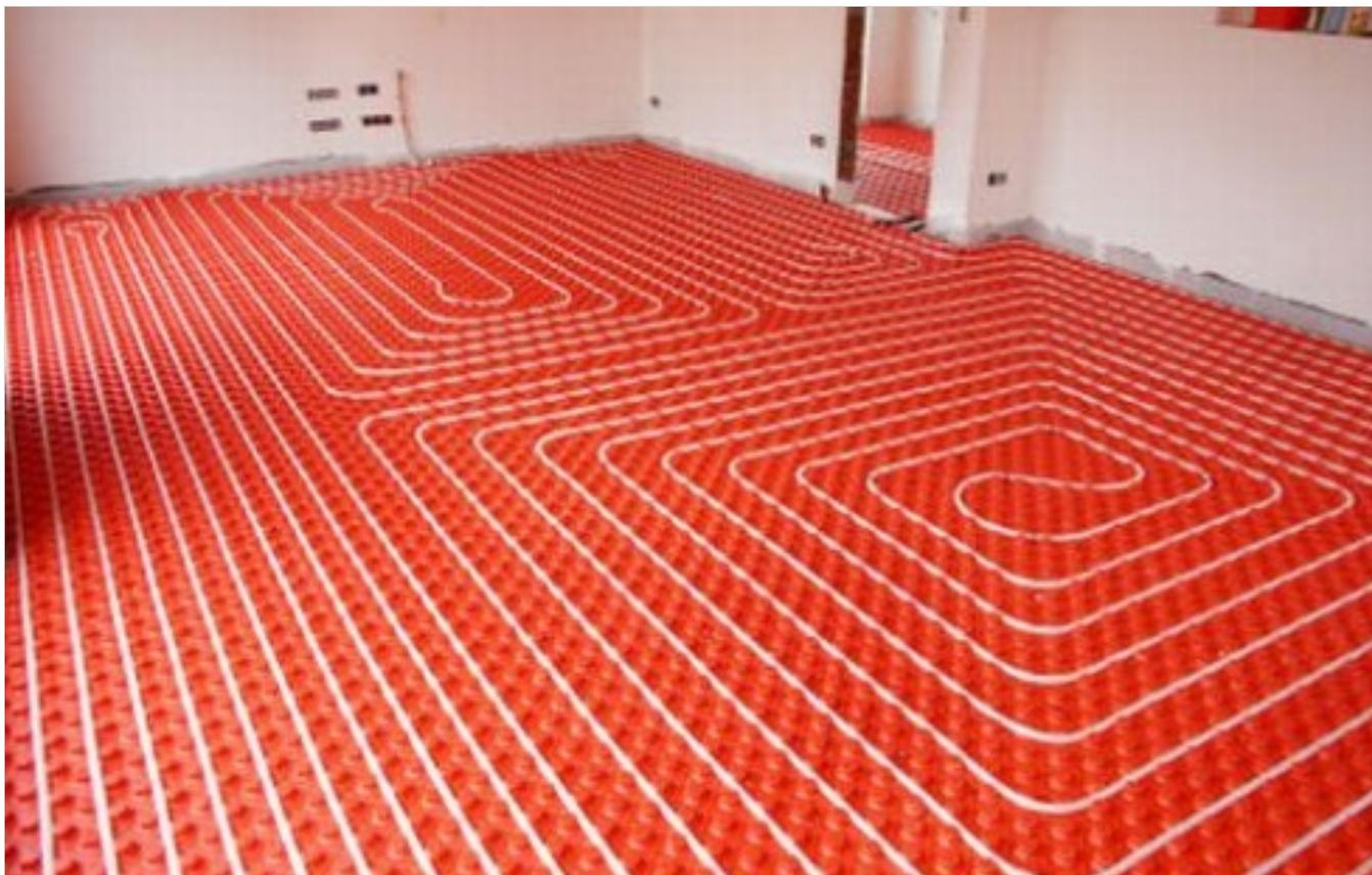
**Pannelli radianti a pavimento Floor radiant panels**
