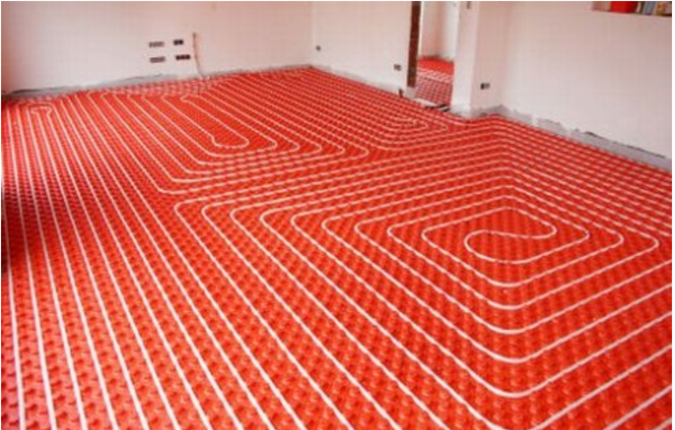
Pannelli radianti a pavimento Floor radiant panels
